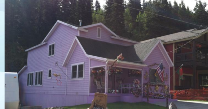
Example of insensitive addition, height should not exceed the primary building
