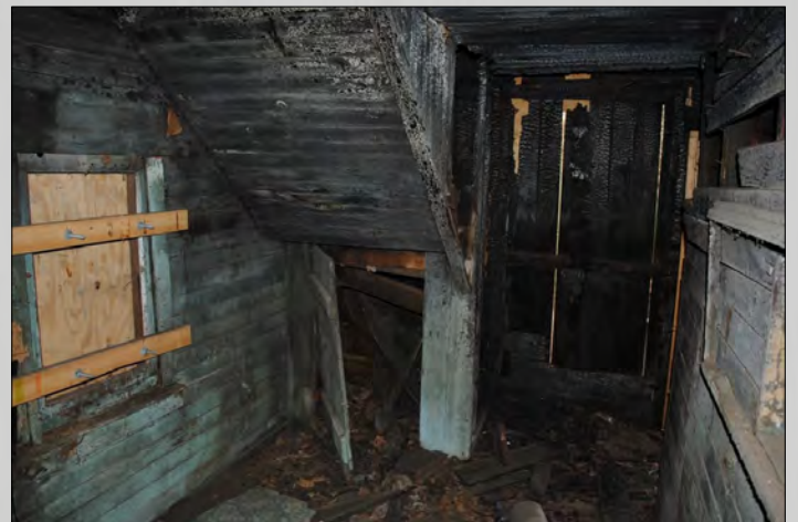
Interior east side "kitchen" view south
