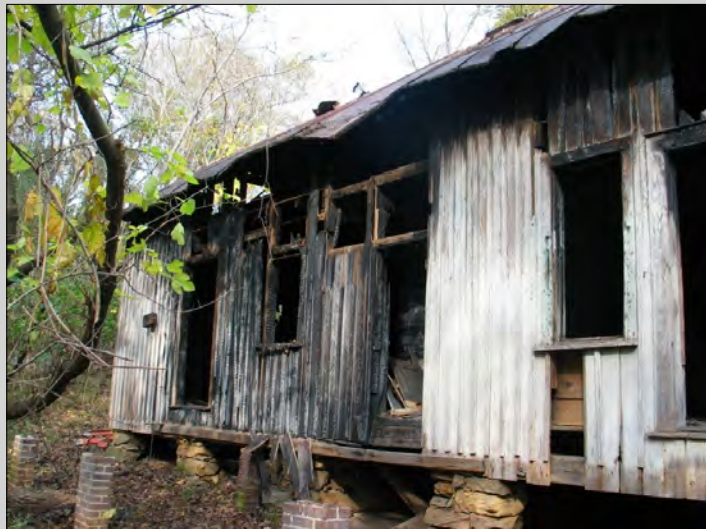
South (front) elevation view northwest
