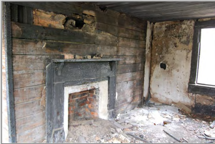
Interior east side view northwest
