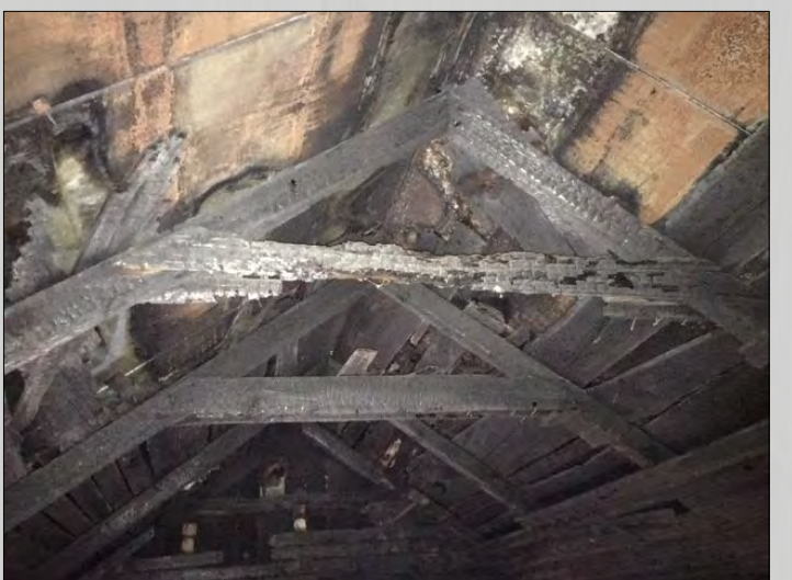
Interior east side loft view west
