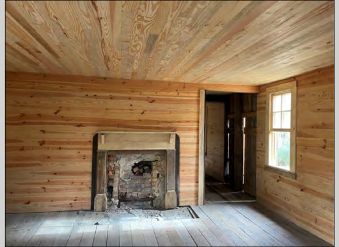
Interior west side view east
