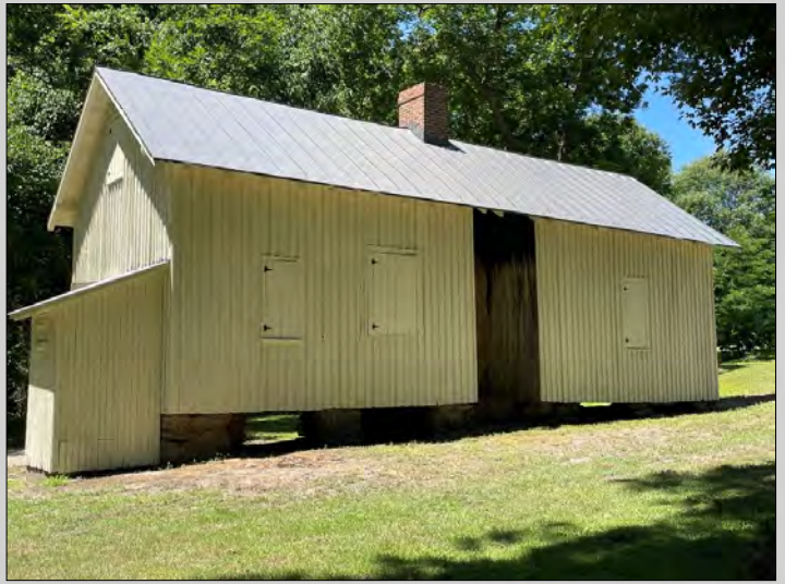
Northeast corner oblique view southwest
