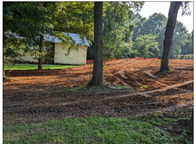
During view looking south from cemetery boundary.
