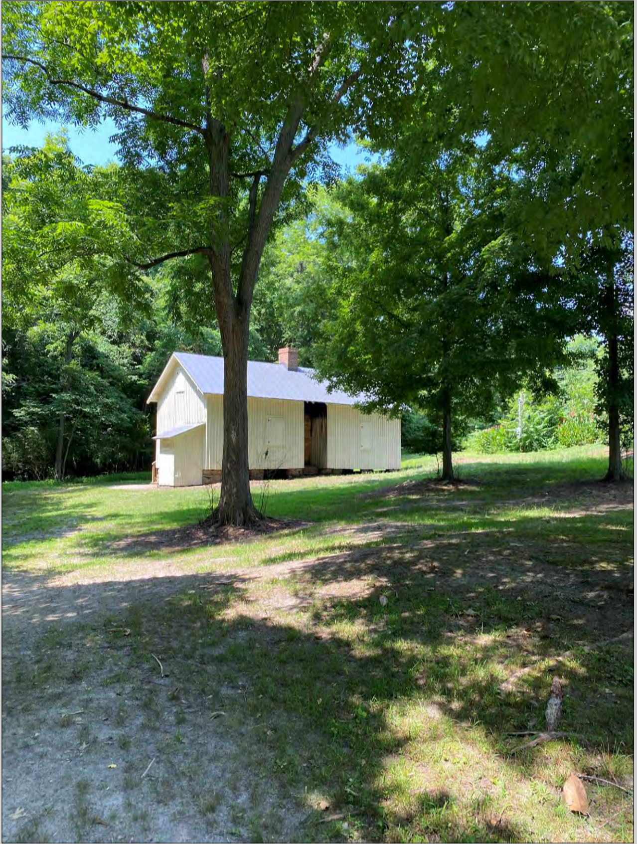
Figure 3. The Ailey Young House after painting in June 2022.
