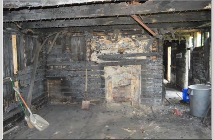
Interior west side view east
