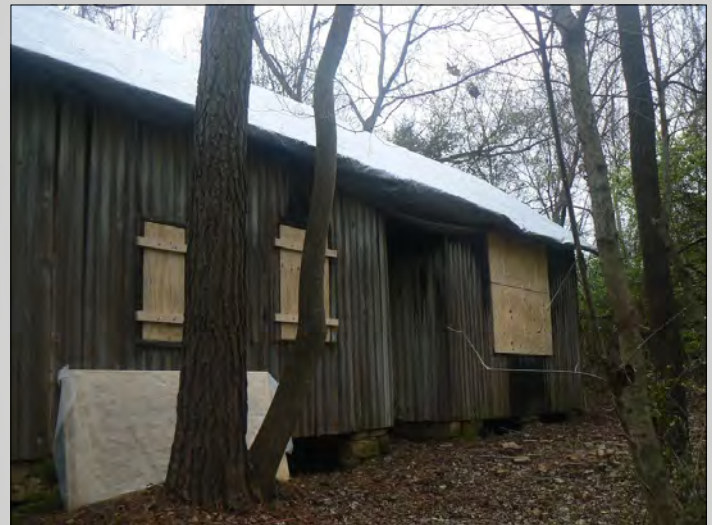
North (rear) elevation view southwest
