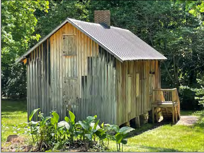
West elevation from N. White Street
