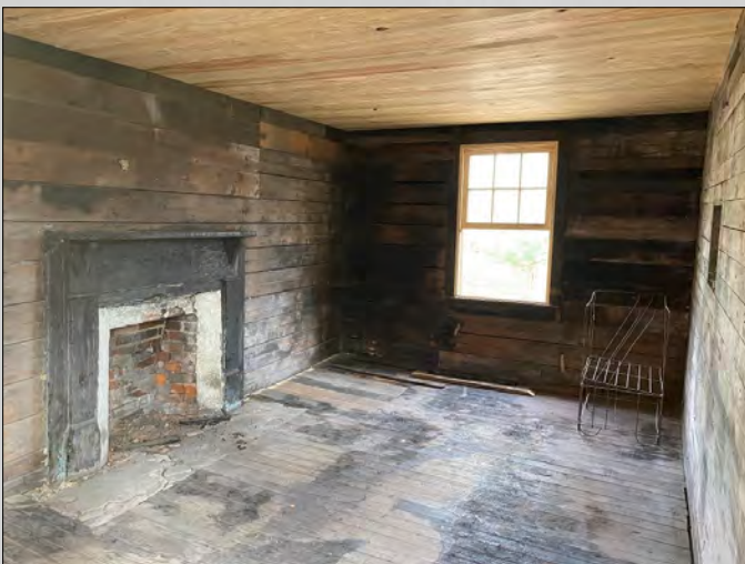
Interior east side view northeast
