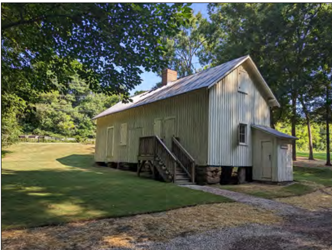
After view looking west from southeast corner of house.
