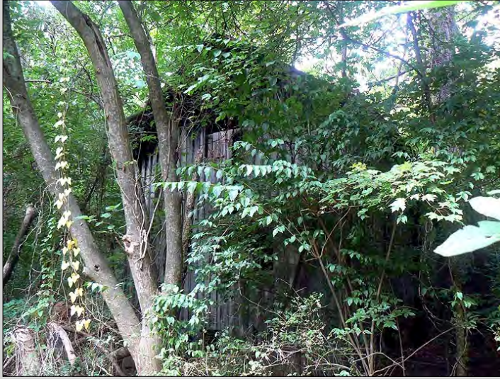
West elevation from N. White Street
