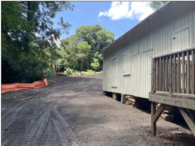
During view looking west at southeast corner of house.
