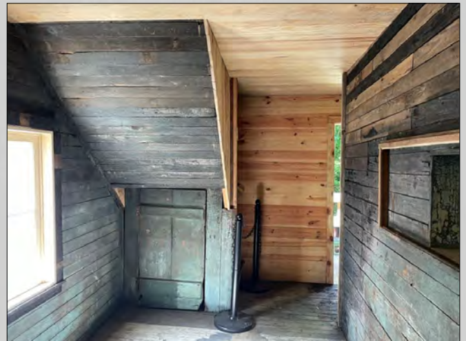
Interior east side "kitchen" view south
