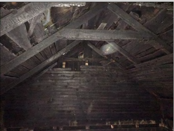
Interior east side loft view west
