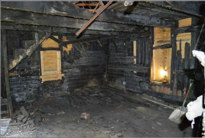
Interior west side view northwest
