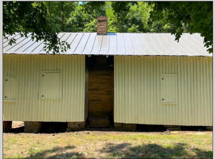
North (rear) elevation view south
