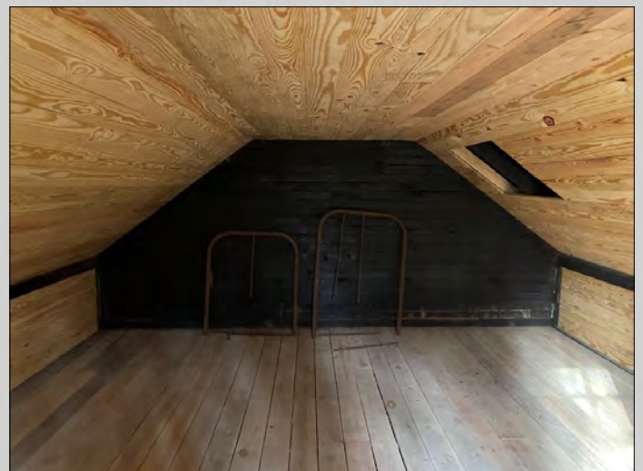
Interior east side loft view west
