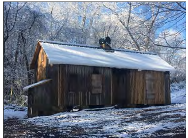
Figure 47. The Ailey Young House in the snow after the roof was completed.
