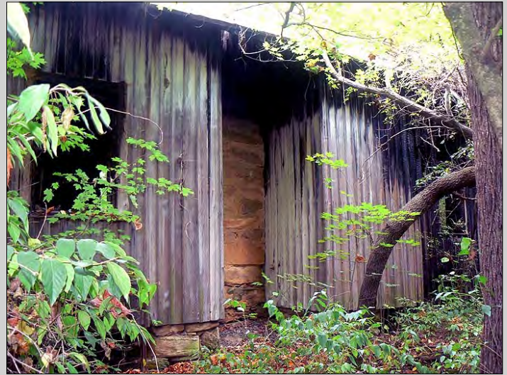
North (rear) elevation view southwest
