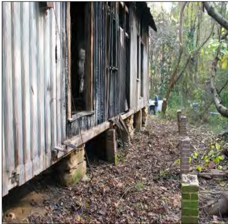
Photograph showing porch piers and floor joists in November 2009
