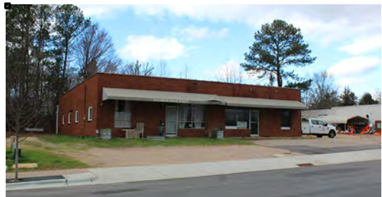
Figure 17: Commercial Building (WA8723) 502-504 South White Street
