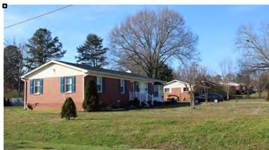
Figure 7: Windsor Park (WA8767) 300-block of Forestville Road
