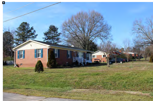
Figure 52: Windsor Park (WA8767) 300 block Forestville Road
