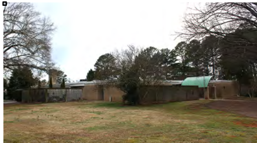
Figure 11: Northern Wake Hospital (WA8705) 250 South Allen Road
