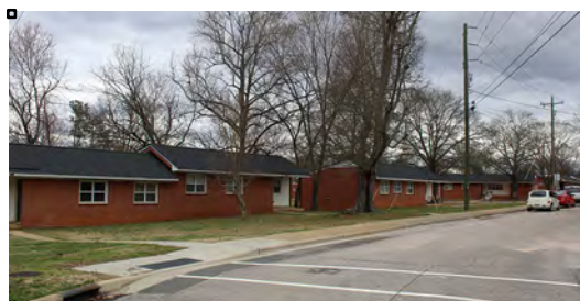
Figure 8: Public Housing (WA8691) 600 North White Street
