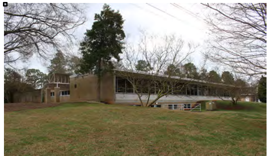
Figure 18: Northern Wake Hospital (WA8705) 250 South Allen Road
