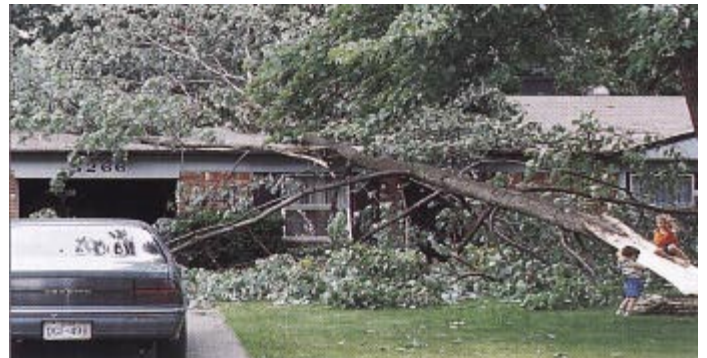
Figure 2. This damage was due to poor tree structure. Cabling would have minimized or avoided the damage.
