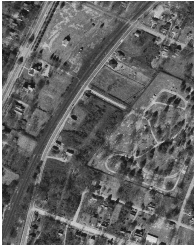
Figure 45: By 1965, only six of the eleven dwellings originally depicted on the 1915 Sanborn map remained standing. By this time, few were still occupied. Two years later, the remainder of these dwellings would be demolished, leaving the Ailey Young House as the sole remaining intact building associated with Simmons Row. Photograph digitized and published by USGS.
