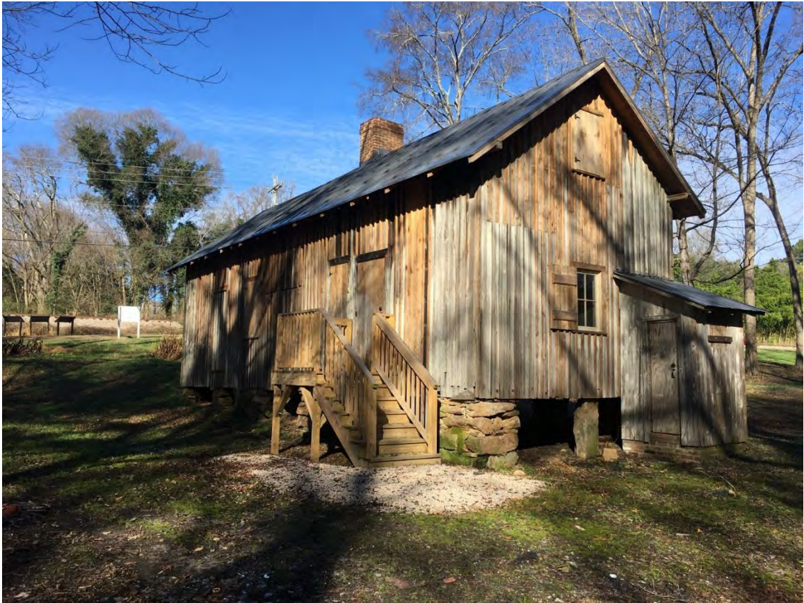
Figure 115: Oblique view of Ailey Young House, south and east façades. Camera facing northwest. Photo by Chris Robey (2021).
