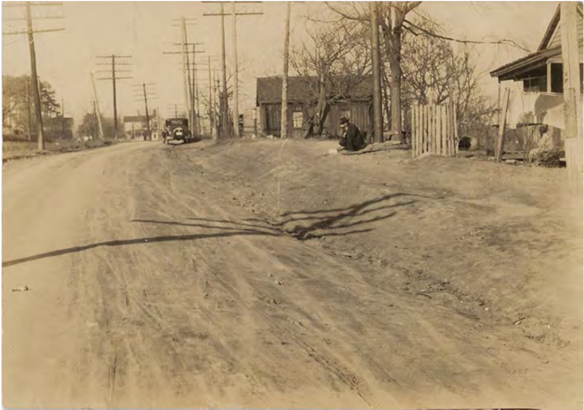
Figure 34: The landscape along Simmons Row was historically much more sparsely vegetated than it is today. In this circa-1930 photograph, the J.B. Carlyle House is visible in the background on the left side of the frame. Today, this house is obscured by a screen of bamboo. Image scanned and published by ZSR Library, Special Collections and Archives.
