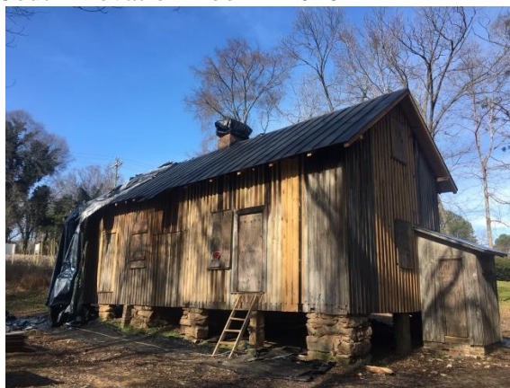
South Elevation Roof in 2020
