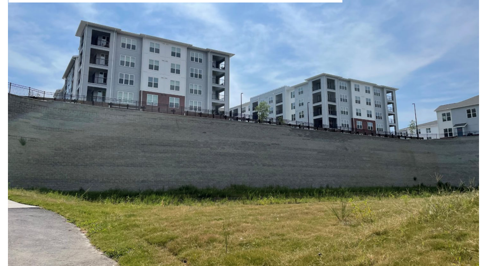
Existing Retaining Wall Example
