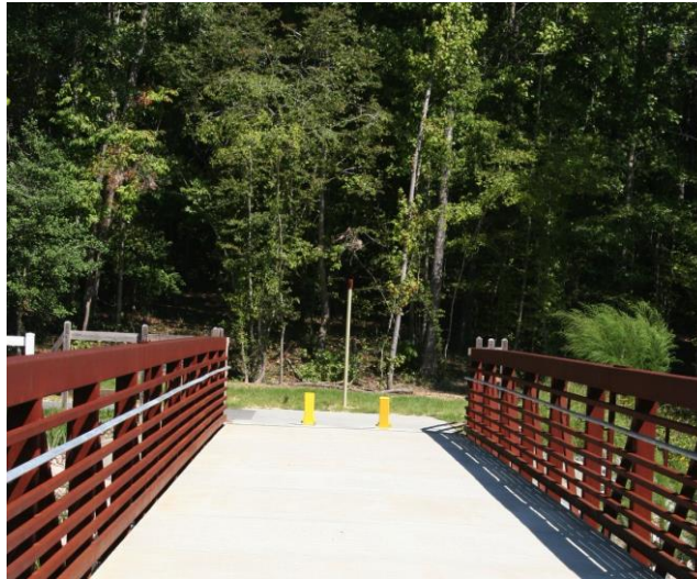
Corten Steel Bridge Over the Neuse River Smith Creek Burlington Mills Greenway
