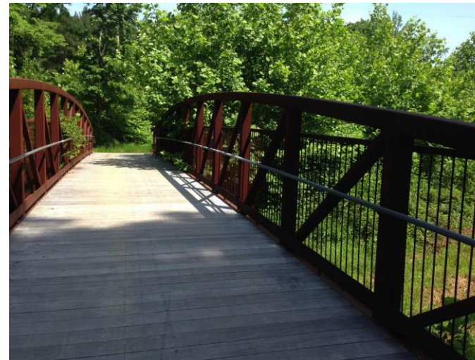
One of Two Corten Steel Bridges Along the Trail
