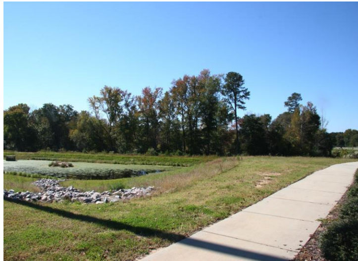
Heritage High Park Pond
