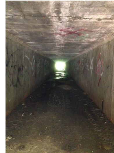
Dunn Creek Pedestrian Underpass Prior to Renovation
