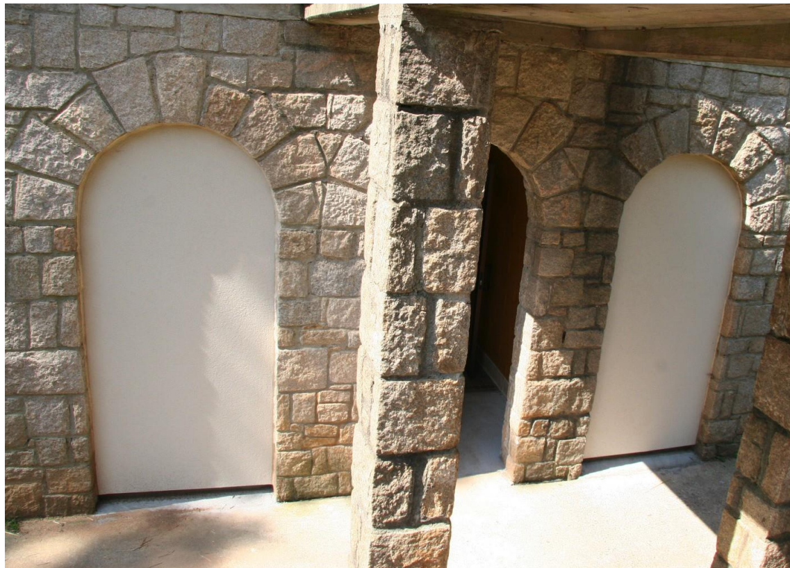
Community House's Plywood-paneled Closed Entryways Holding Park
