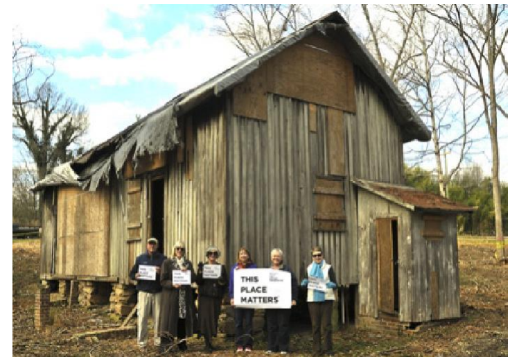
Ailey Young House Discovered During Historic Building Survey 2008
