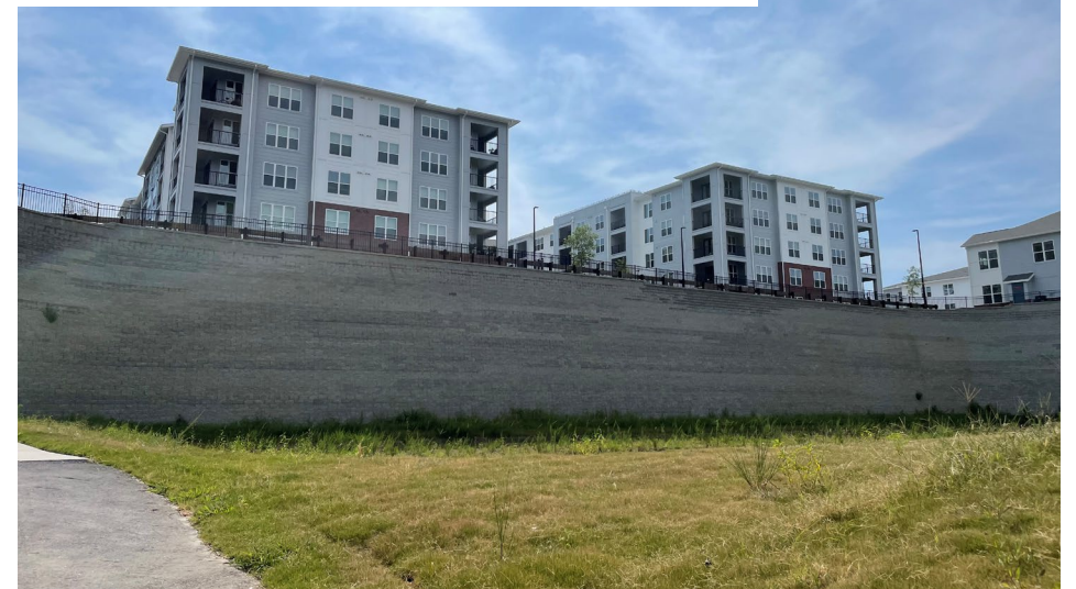
Existing Retaining Wall Example
