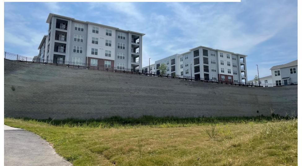
Existing Retaining Wall Example
