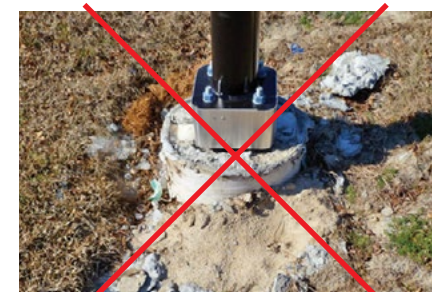
NOT Acceptable Footer Detail
