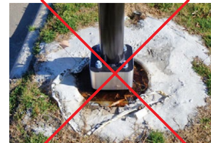
NOT Acceptable Footer Detail
