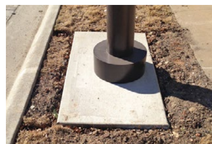
Acceptable Footer Detail
