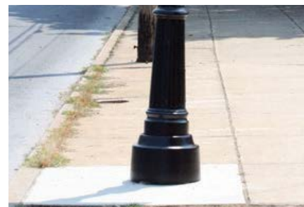
Acceptable Footer Detail
