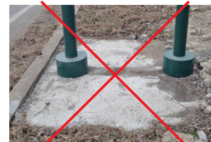
NOT Acceptable Footer Detail
